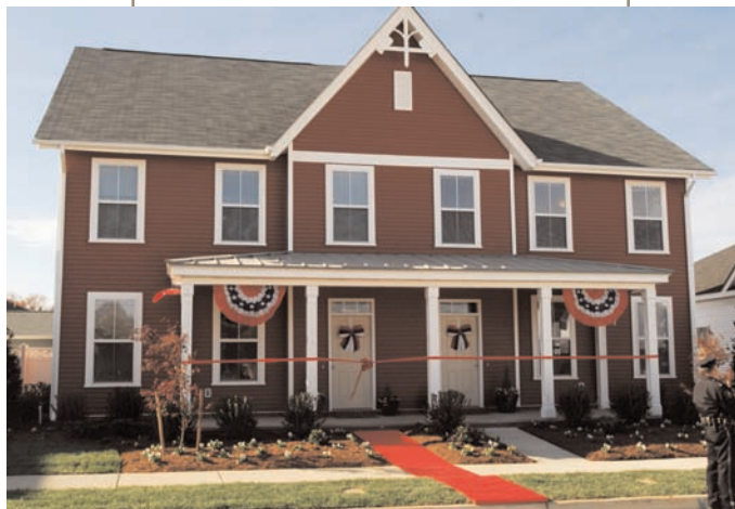
A new home at the Village at Whitehurst in Norfolk, Va., managed by Lincoln military housing. U.S. Navy photo by Mass Communication Specialist 2nd Class Kevin L. Burluson
