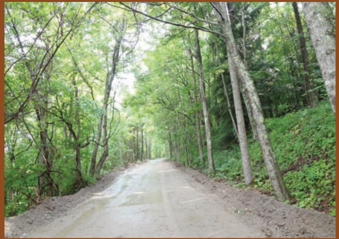
The same road after the improvements. Photo courtesy of the JTF Summit Staff
