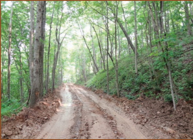
Before road improvement by the IRT program at the Summit. Photo courtesy of the JTF Summit Staff
