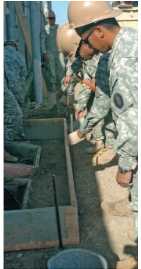
Hawaii Army National Guard soldiers from the 230th Engineer Company, cut wood to build forms that will surround the electrical boxes and protect them from increased damage, during an Operation JUMP START mission along the California/Mexican border in April. Operation JUMP START is a federal initiative which uses the National Guard to give support to the U.S. Customs & Border Patrol in securing the southwestern border. Hawaii engineers were attached to Task Force STEEL CASTLE, the engineering slice of the California National Guard's OJS mission.
